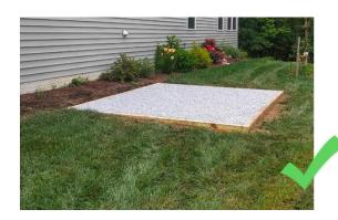
Framed in crushed stone. Stones must fill to the top of the frame.
